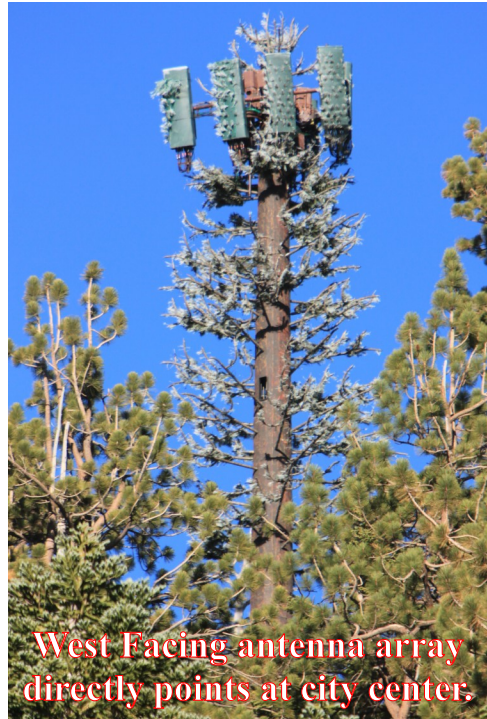
Angel's Roost Macro Tower antennas with faux plastic needles.
