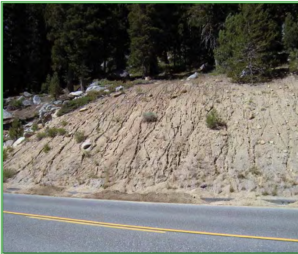
Figure 3.3: This road cut photo illustrates lack of cover and infiltration capacity and resulting runoff.
