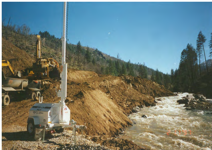
Figure 3.2: This photo of the American River shows a mass failure that blocked the river for some period of time. This slide is believed to be the result of lack of vegetation from a previous fire and defoliation efforts and from water associated with a 100 year precipitation event (1997)
