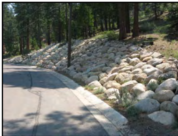
Riprap Slope Stabilization: Good example
