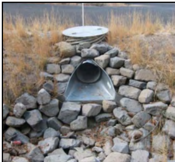
Drainage Outlet: This one is outlet from a basin
