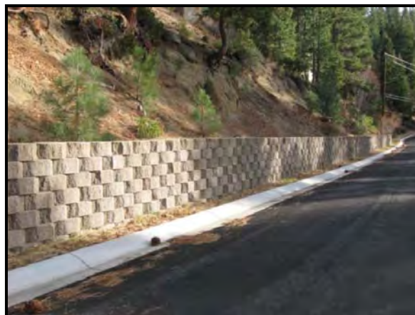
Retaining Wall: Block structure in good condition.
