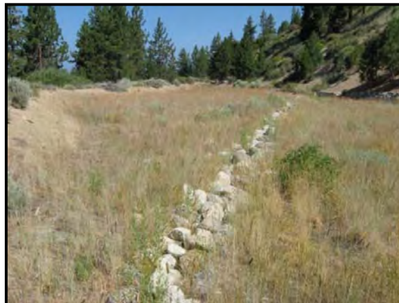
Bed Filter: This basin looks like a dry basin but has an underdrain to carry flows back to the surface
