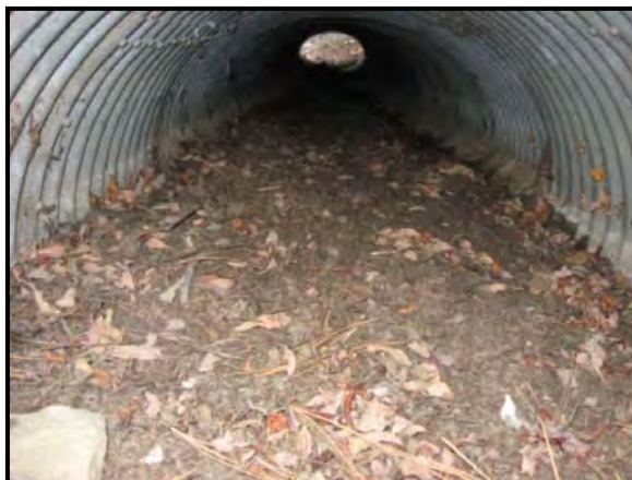
Conveyance Piping: Example of need for cleaning
