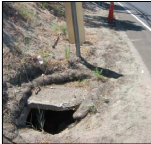
Drainage Inlet: Needs improvements
