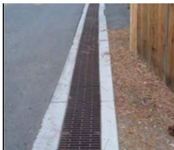
Drainage Inlet: includes slotted drains
