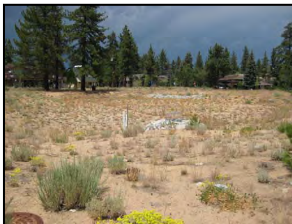
Dry Basin: This basin has an outlet to control sedimentation and a gauge to measure depth of sediment accumulation
