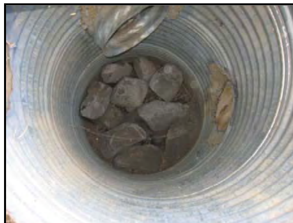
Drainage Inlet: typical with rock bottom
