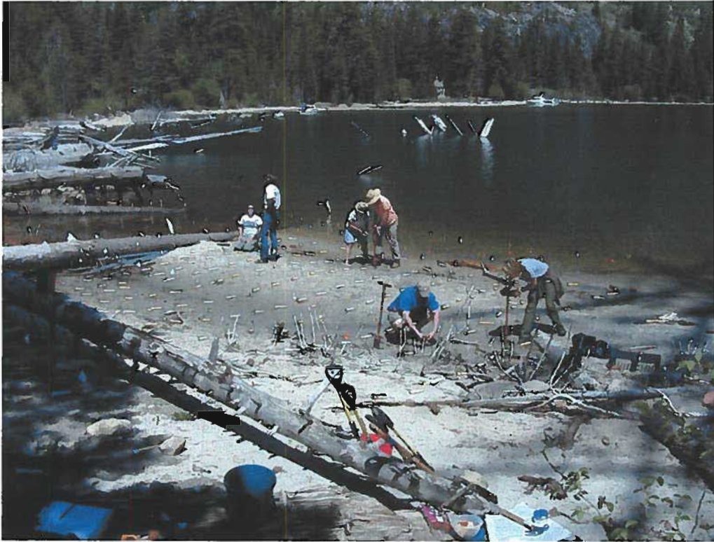
Photo 3. CDPR crew installing TYC at Avalanche beach, June 2003.
