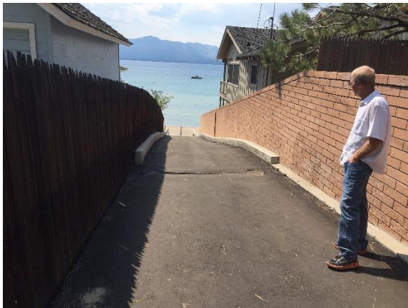
Photo Set 2: The runoff takes a turn from Tallac Dr. and flows down an old boat ramp directly into Lake Tahoe. As a result, sand is eroded away.
