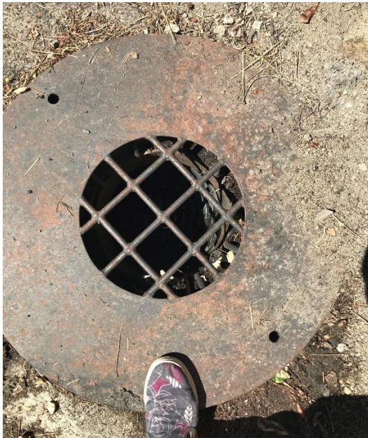
Photo Set 4: Stormwater infrastructure installed in the 70s is out of date or undersized. Left photo – a typical drainage inlet in the steep neighborhood of Zephyr Heights. The project could update these to improve capture. Right: Basin installed during PineWild development never drains and is in a riparian zone. Relocation options exist.
