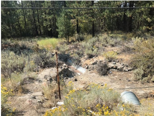
Photo Set 5: Outfalls from US-50 uphill of Bourne Meadows lack treatment and go straight to McFaul Creek. Left Photo: this is the location of the proposed large basin. Right Photo: Just south of the outfall pictured on the left, this highway outfall can also be routed to the new basin.
