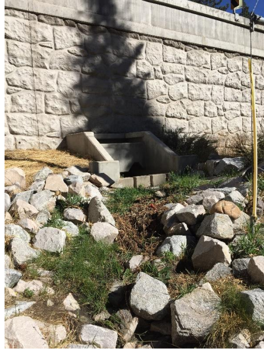
Photo Set 1: Runoff from Catchment 4 (Zephyr Heights) is routed beneath the highway onto Tallac Dr. in Marla Bay. The channel and vaults along its path could be retrofit to provide treatment or infiltration.
