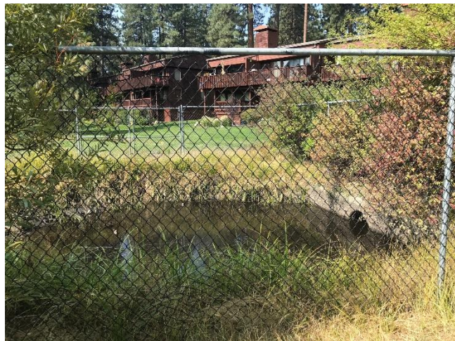
Photo Set 4: Stormwater infrastructure installed in the 70s is out of date or undersized. Left photo – a typical drainage inlet in the steep neighborhood of Zephyr Heights. The project could update these to improve capture. Right: Basin installed during PineWild development never drains and is in a riparian zone. Relocation options exist.
