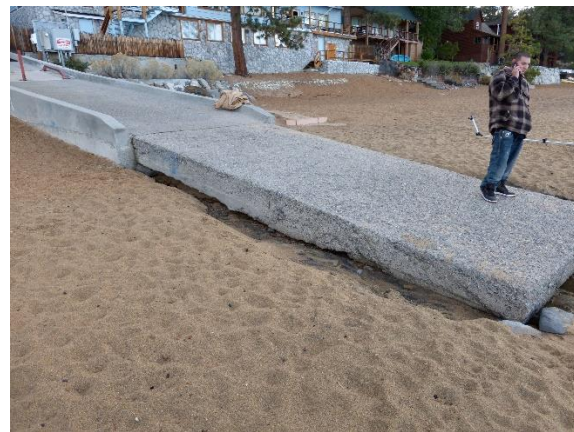
Photo Set 2: The runoff takes a turn from Tallac Dr. and flows down an old boat ramp directly into Lake Tahoe. As a result, sand is eroded away.
