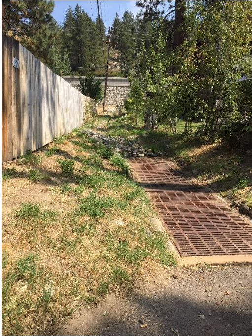
Photo Set 1: Runoff from Catchment 4 (Zephyr Heights) is routed beneath the highway onto Tallac Dr. in Marla Bay. The channel and vaults along its path could be retrofit to provide treatment or infiltration.
