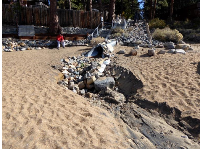
Photo Set 3: A second outfall in Marla Bay at the end of Lakeshore Drive receives runoff from catchments 1, 2a, and 2b with little treatment and discharges directly to the Lake. Runoff from 1 and 2b would be re-routed to the new treatment basin near Bourne Meadows. The existing rock ditch and vaults could be retrofit to treat runoff from 2a prior to discharging to the Lake.
