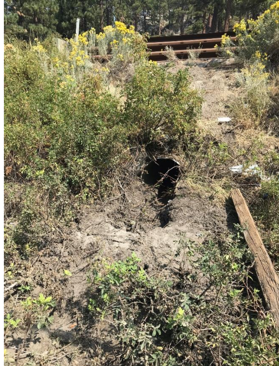
Photo Set 5: Outfalls from US-50 uphill of Bourne Meadows lack treatment and go straight to McFaul Creek. Left Photo: this is the location of the proposed large basin. Right Photo: Just south of the outfall pictured on the left, this highway outfall can also be routed to the new basin.
