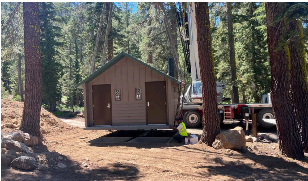
New bathroom installed at Watson Lake August 2023
